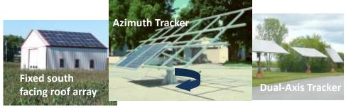
components that are cycling more often. Compared this to a simpler Azimuth Drive tracker with fewer moving parts, fewer sensors and fewer operating cycles. Azimuth drive trackers also generally use less energy.
