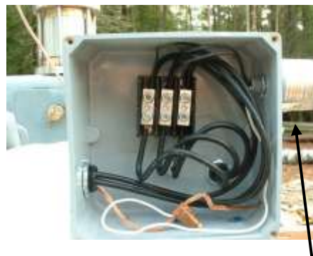
Lightning Arrester
