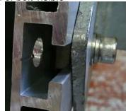
**CORRECT BOLT M8x20mm** Space between bolt and rail when torqued
